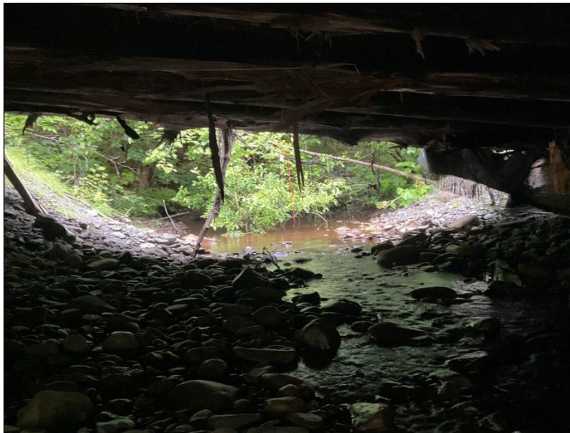
Figure 3.—Looking under bridge, downstream at waypoint 631.
